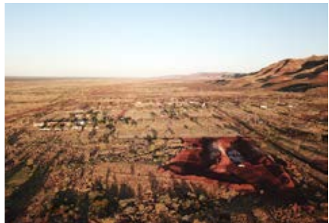
Demolition started recently, with all material to be buried onsite.
