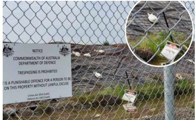
Large mounds of contaminated dirt have been stockpiled next to the quarantine centre at Pinkenba.
