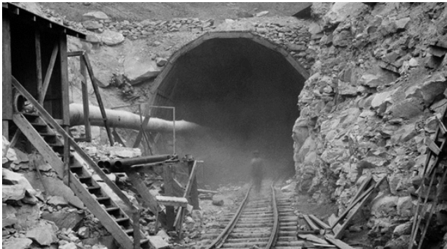
In the photo above, dust circles a worker during the construction of the Hawks Nest Tunnel in 1930. Workers on the project were exposed to toxic levels of silica dust; hundreds ultimately died. Courtesy of Elkem Metals Collection, West Virginia State Archives
