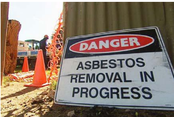
While the ACT Government committed $1 billion to buy and bulldoze affected homes, it made no provision for residents who contracted mesothelioma.
