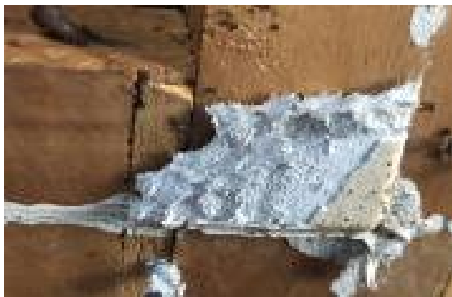
LDB ceiling sheet torn from the ceiling battens. The corner of the sheeting remains attached with a flex sheet nail. Torn is an apt descriptor because LDB tears like cardboard.
